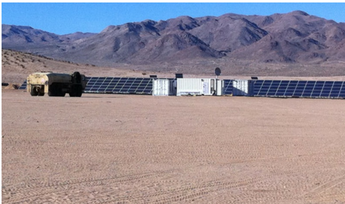
Example of a 1-megawatt "microgrid" currently in use by the US Army
