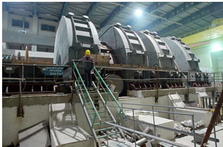
The Bushehr nuclear power plant
