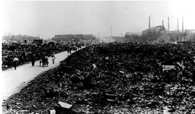
Nagasaki's Iwakawa-machi neighborhood in ruins. Photograph by Ogawa Torahiko
