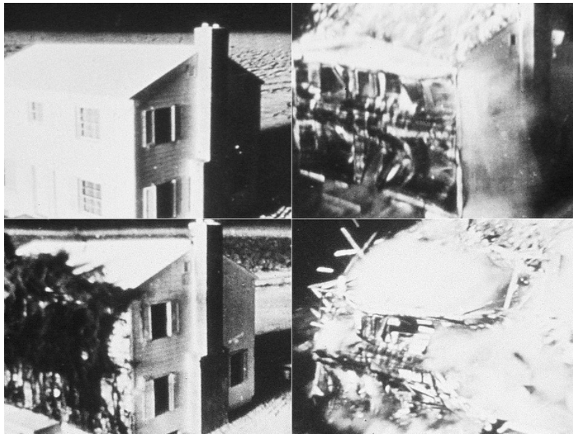
Figure 2. Damage done by 5 psi on a house
