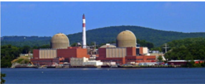
Indian Point Nuclear Power Plant
