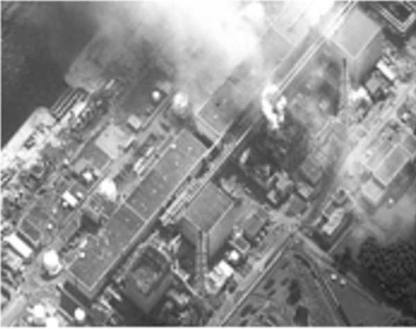
Hydrogen Gas Explosion
