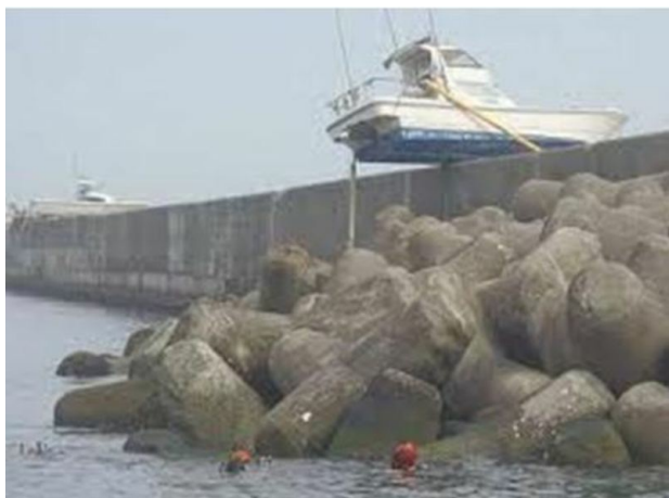
In Tohoku, seawalls and tetrapods were overwhelmed
