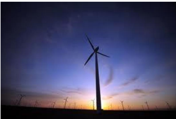
Wind turbines in Gansu
