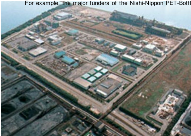
Kitakyushu's eco-town under construction
