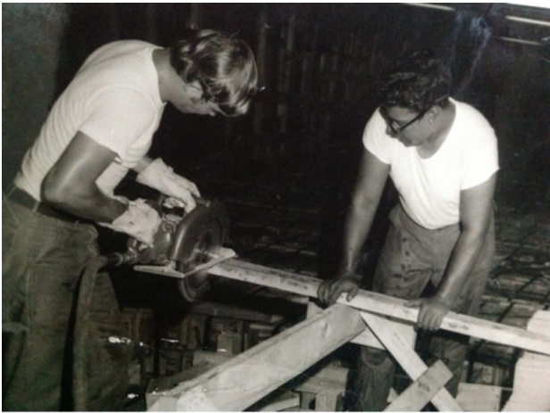
U.S. service members work beneath decks ensuring the chemical weapons fit snugly together. Tim Gravely
