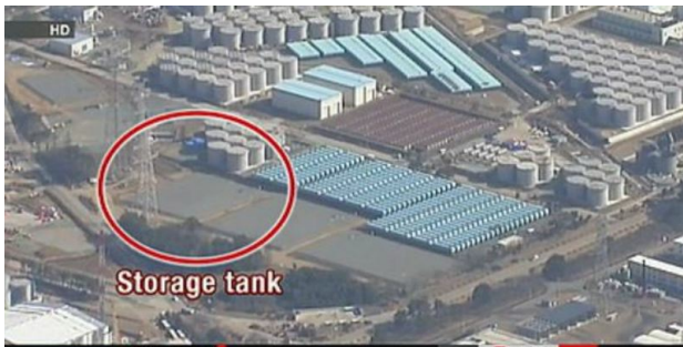
Leaking storage tank and TEPCO attempts to contain contaminated water at Fukushima Daiichi (NHK)
